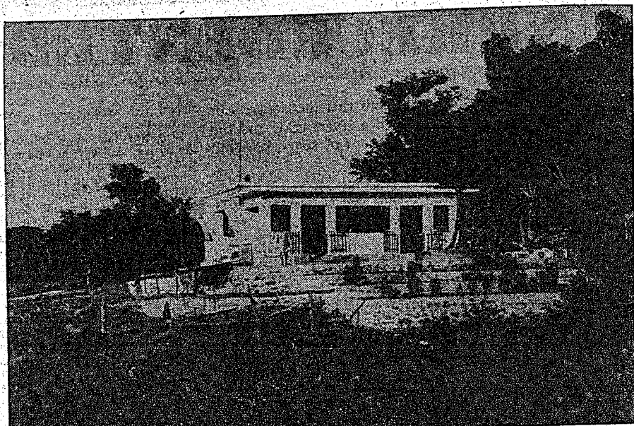
The Haludpukur Holiday Home of the Reserve Bank Employees' Association, Calcutta. It has two family units
