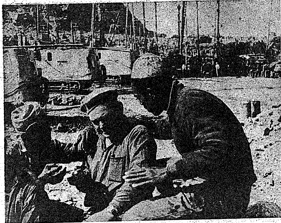
At the Aswan Dam construction site, a Soviet engineer guides UAR workers.
