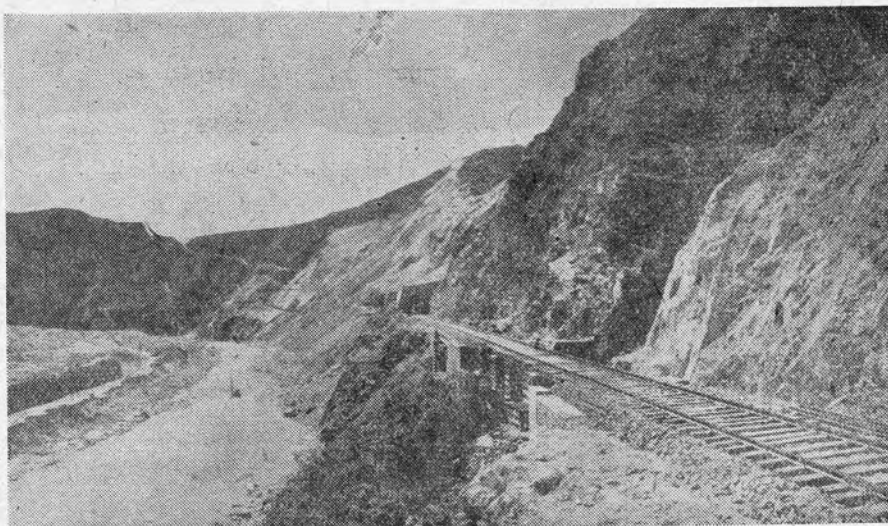
The Tienshui-Lanchow railway runs through tunnels totalling 10 km. in length
