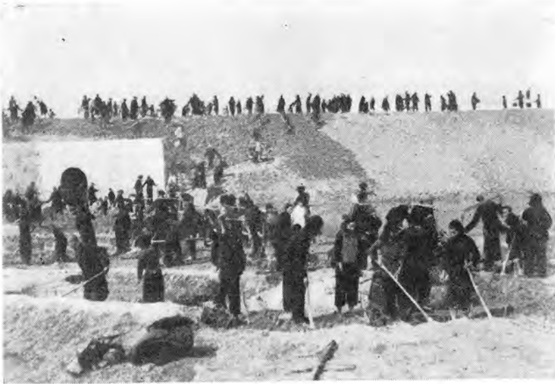
Mutual aid teams re-enforce neglected river embankments to protect their land against flood.
