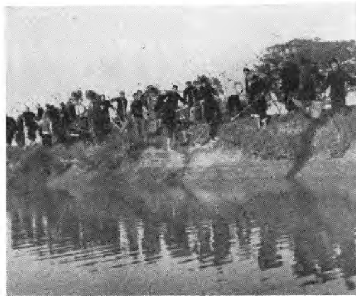
To irrigate their land, peasants volunteer enthusiastically to repair a reservoir.
