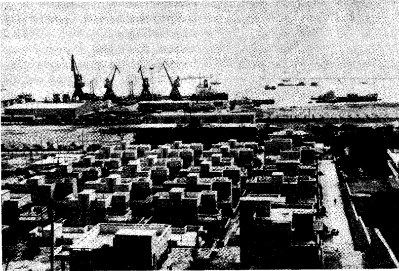
The 20,000-ton-class deep-water wharf in Shenzhen's Chiwan Harbour.
