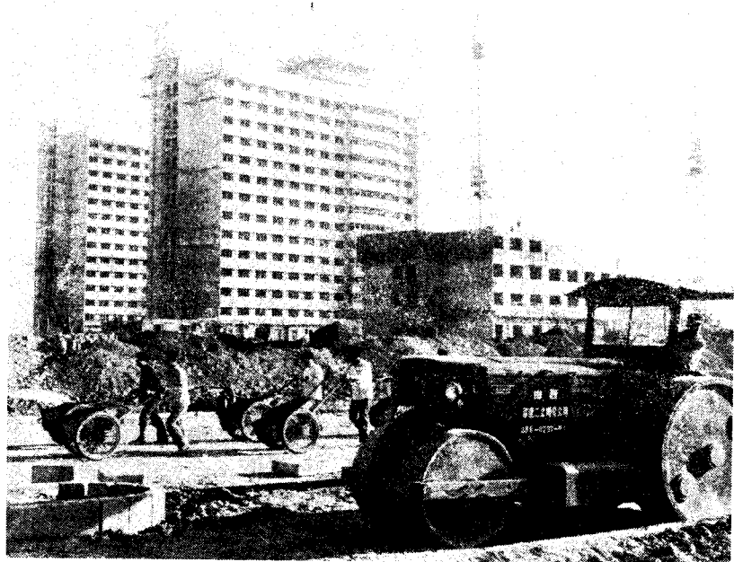
Sino-American jointly built living quarters at the Pingshuo Mine.
