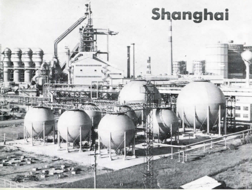
The No.1 Blast Furnace of the Shanghai Baoshan Iron and Steel Complex and its conveyance system were completed recently. Most of the equipment was imported from Japan.
