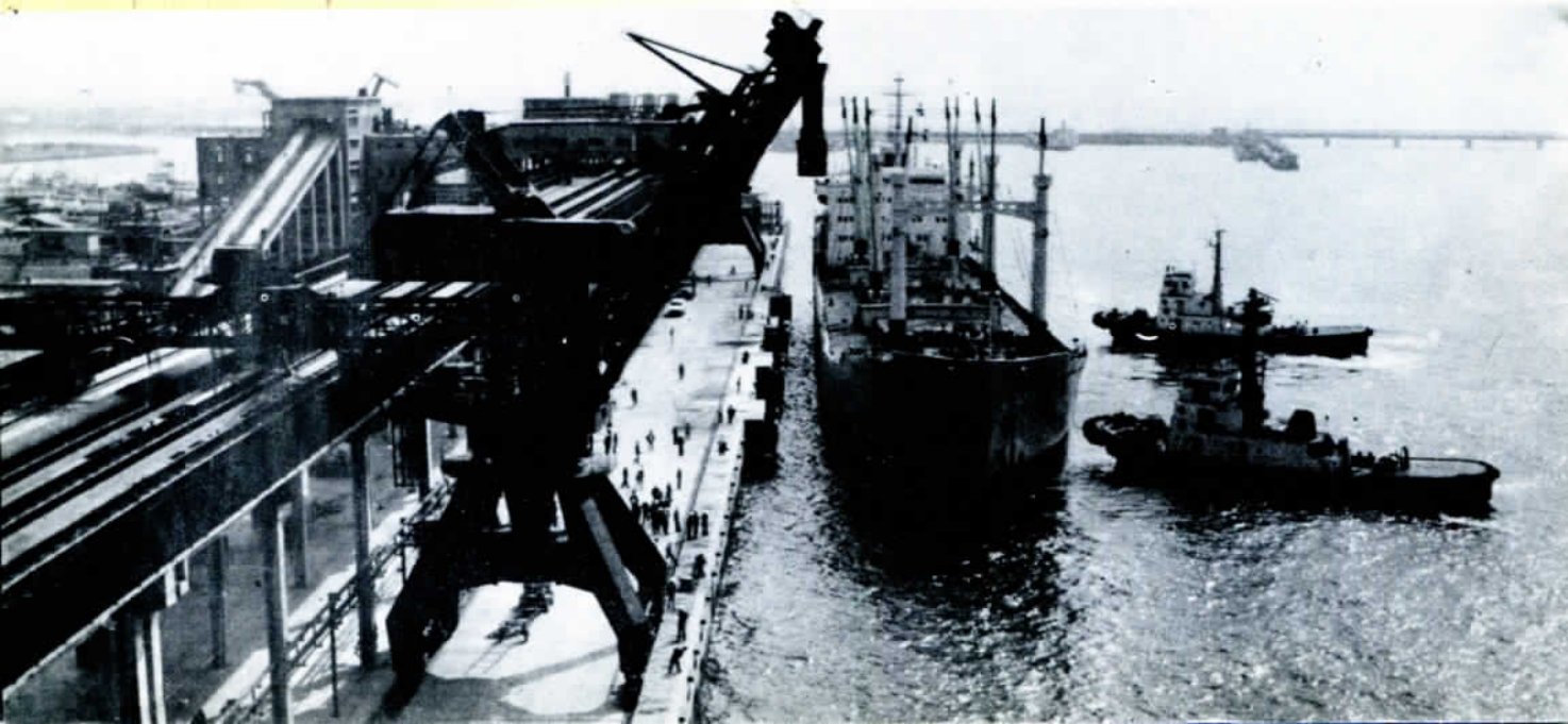
A special dock for shipping coal in Qinhuangdao.
