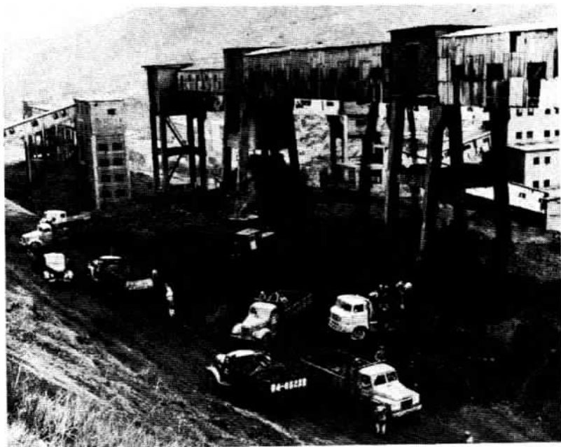
A worksite in the Duerping Coal Mine in Xishan, Shanxi Province.
