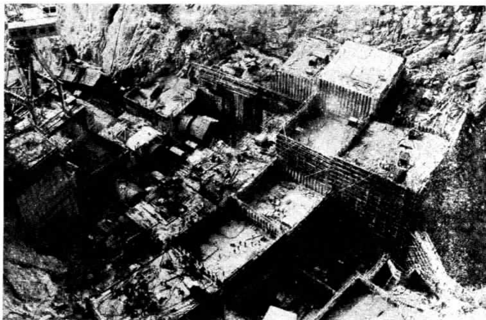
The gigantic Longyang Gorge Hydroelectric Power Station under construction.
