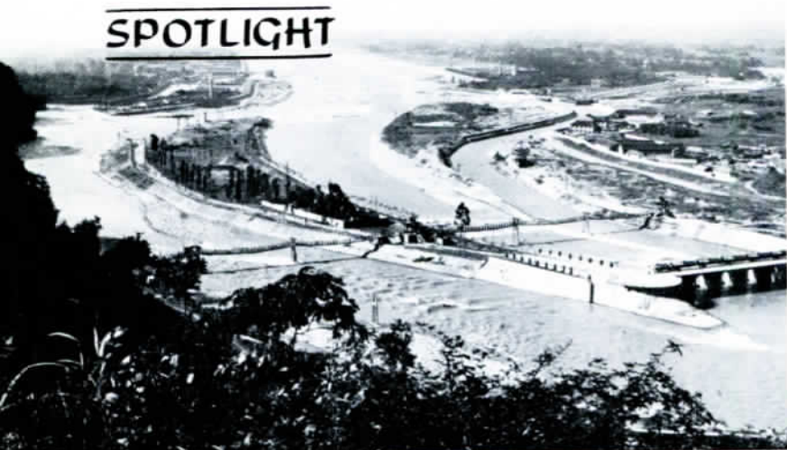
A bird's-eye view of the Dujiang Water Control Complex.
