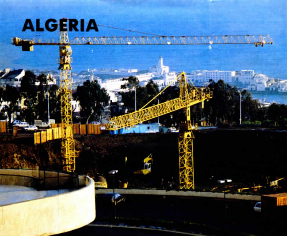
A construction site in Algiers.
