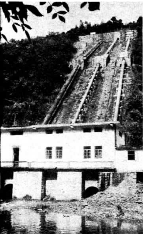
The Daqiao Hydropower Station in Guangdong's Longmen County.
