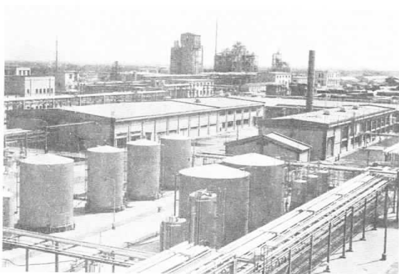
The Yantai Synthetic Leather Factory in Shandong, one of last year's 70 key construction projects, now completed.
