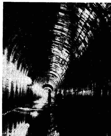
The tunnel of the Tianjin water diversion project, 12.3 kilometres long, 5.7 metres wide and 6.25 metres high, is the biggest of its kind in China.
