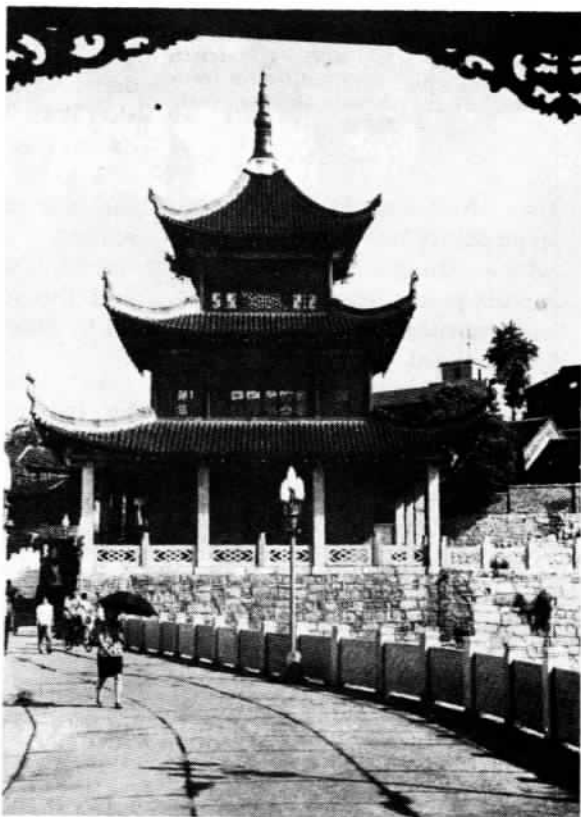
Repairs saved Jiaxiu Pavilion—a famous ancient building (built in 1597) in Guiyang, Guizhou Province.
