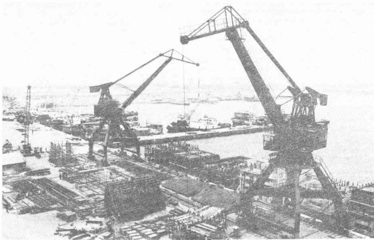
A coal dock in Qiphuangdao under construction.
