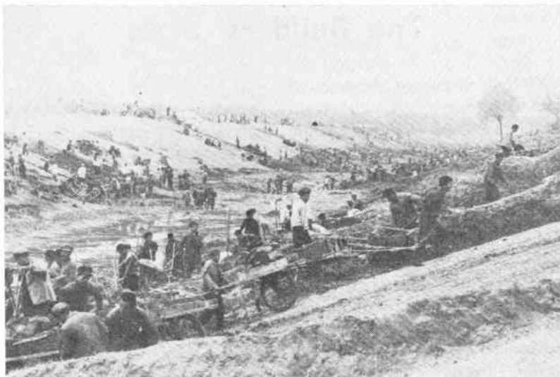
Working for the Panzhuang water-diversion canal project in Shandong.
