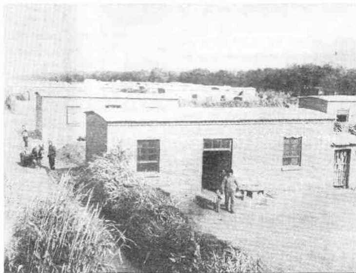
New houses for Shandong's Taiping Village residents whose former homes were dismantled to make room for the construction project.
