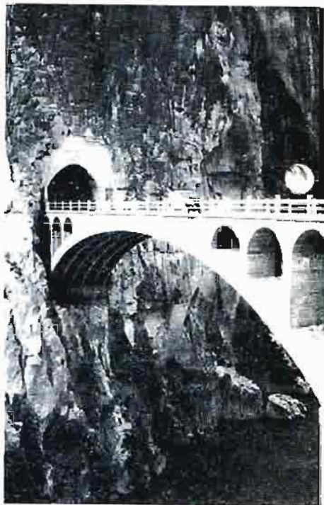
A single span double-arch bridge across the Nujiang River on the Sichuan-Tibet highway.
