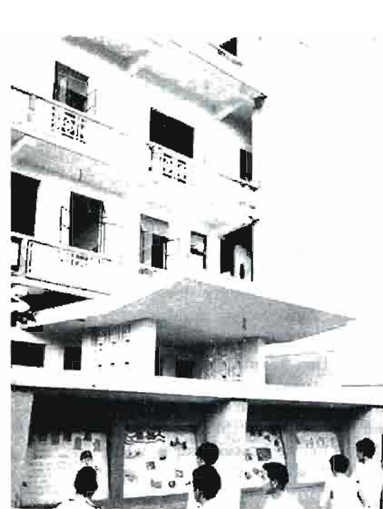
Cultural centre of a commune in Jiangsu Province.
