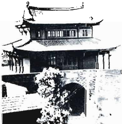
Newly renovated Qiyimen (Uprising Gate) in Wuchang.
