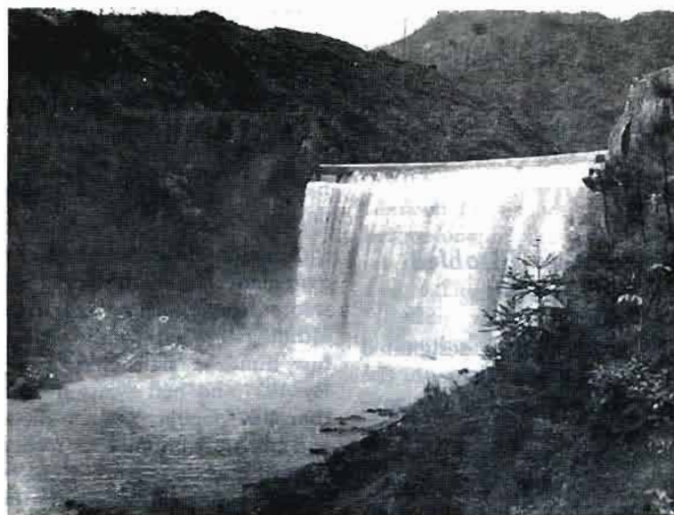
Reservoir spillway of the Panxi hydropower station in Jinyun County, Zbejiang Province.
