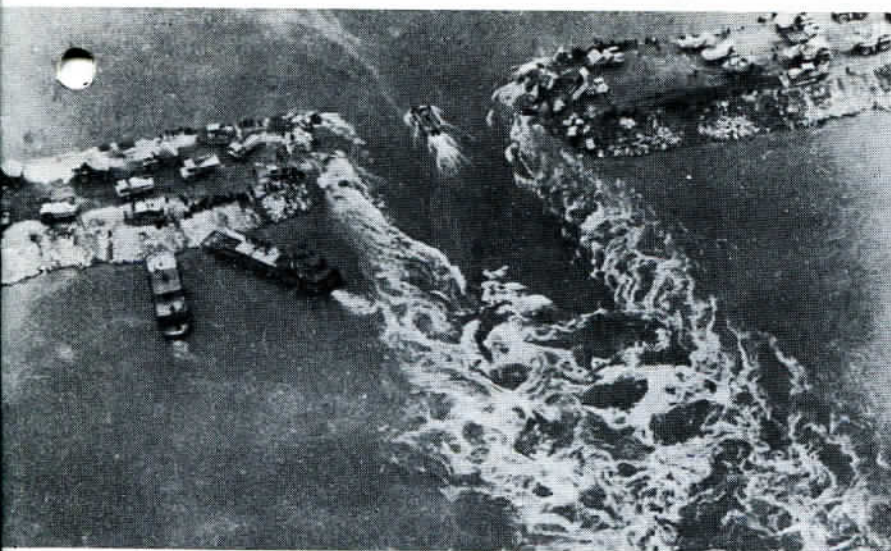
The cofferdam at Gezhouba.
