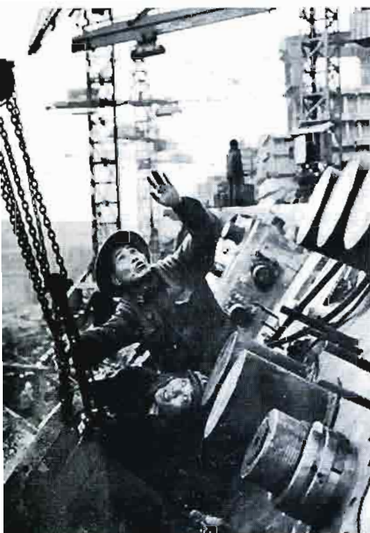
At work on the Gezhouba Water Conservancy Project.
