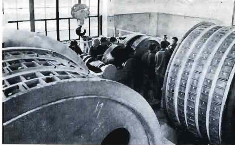
Installing a large winder for a shaft.
