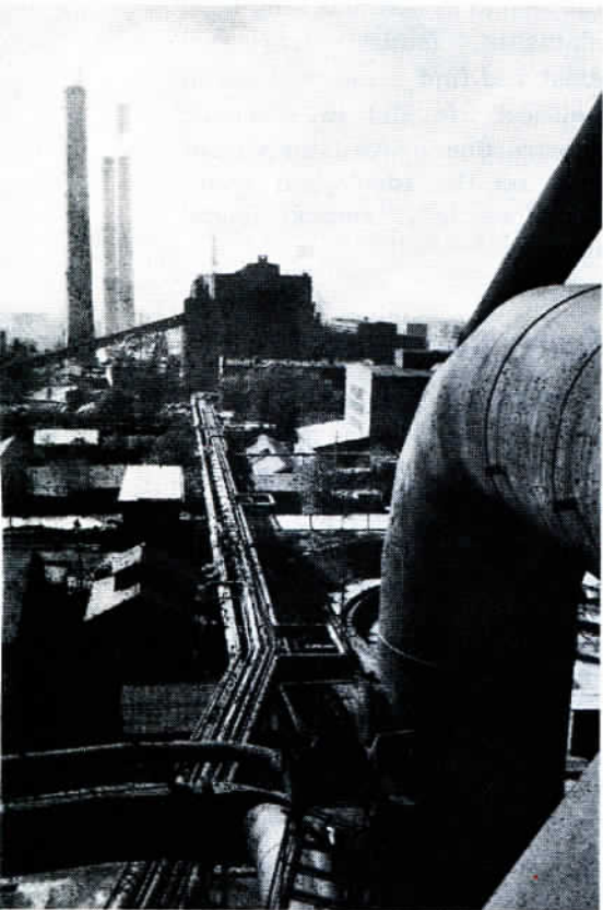
Waste gas from blast furnaces and coke ovens in the Wuhan Iron and Steel Company, central China, is piped to a thermal power station.
