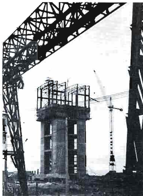
A headframe under construction in the Huainan Coal Mine.
