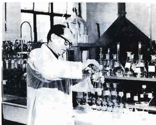
Dong Zicheng making chemical analysis of the electroplating fluid.
