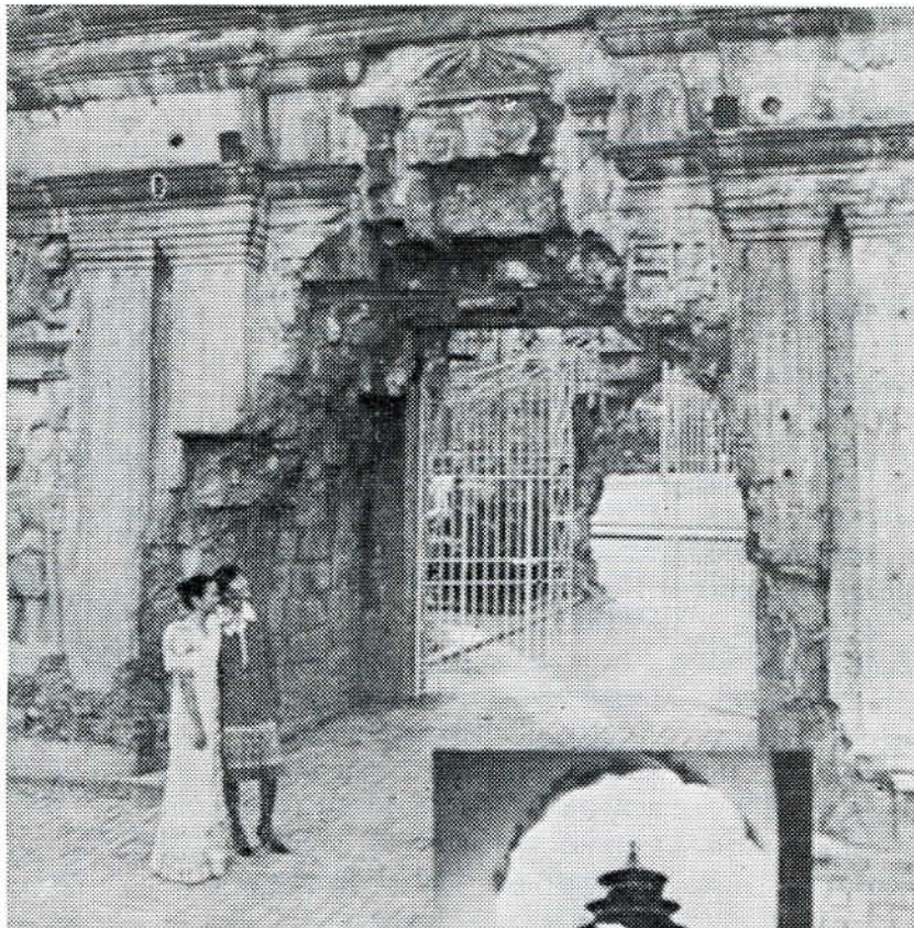
Main Gate, Fort Santiago, Intramuros, Manila.
