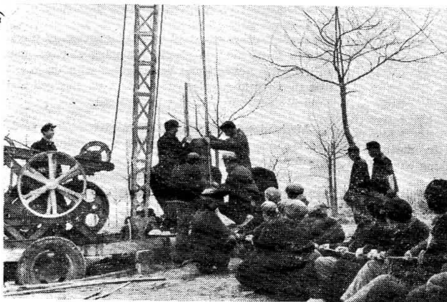
Working together in sinking a power-operated well.
