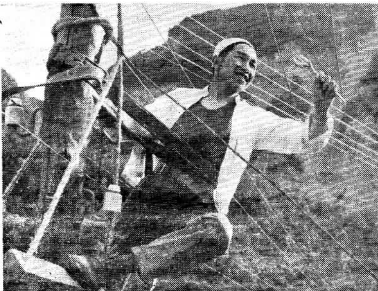
A peasant electrician putting up transmission lines in northwest China's Ningsia.
