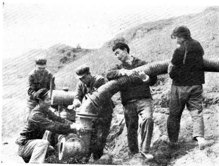
P.L.A. men help a production brigade install a pump.
