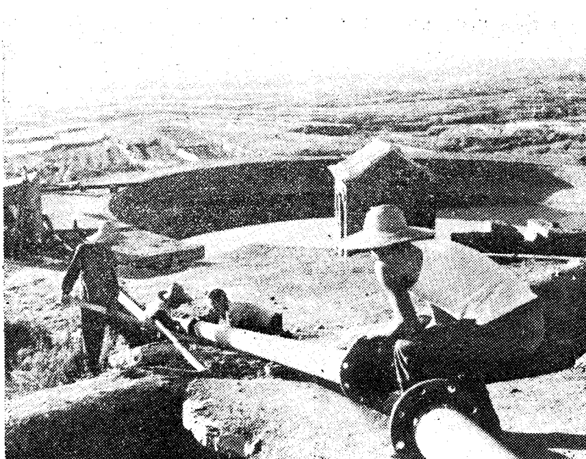
Laying a pipeline to conduct water up the hills in Hsiyang.
