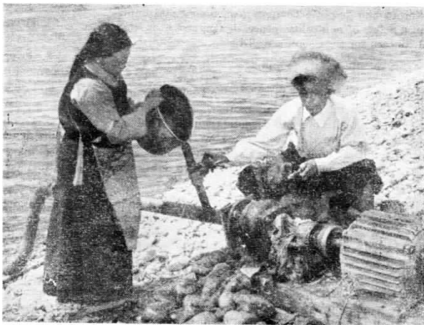
Working an electric pump near Lhasa
