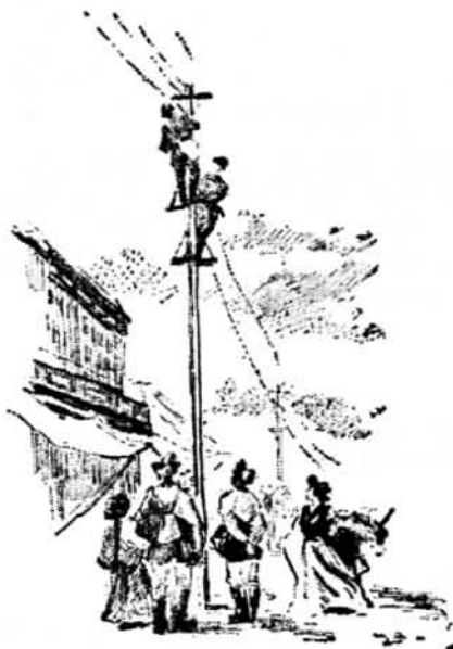
Putting Up Power Lines
