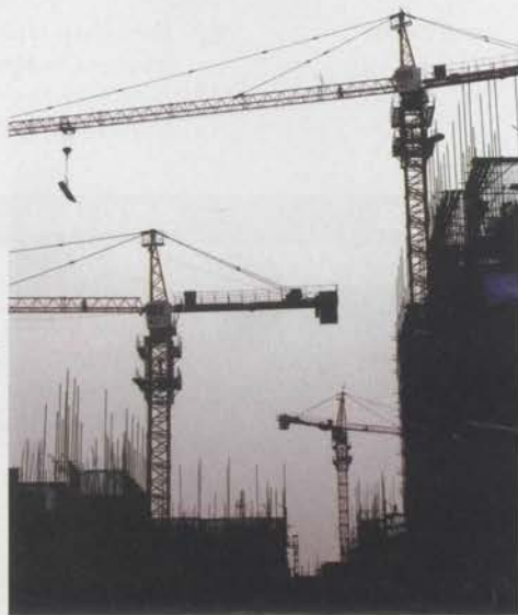
New construction in Shaoyang City, Hunan Province. IC
