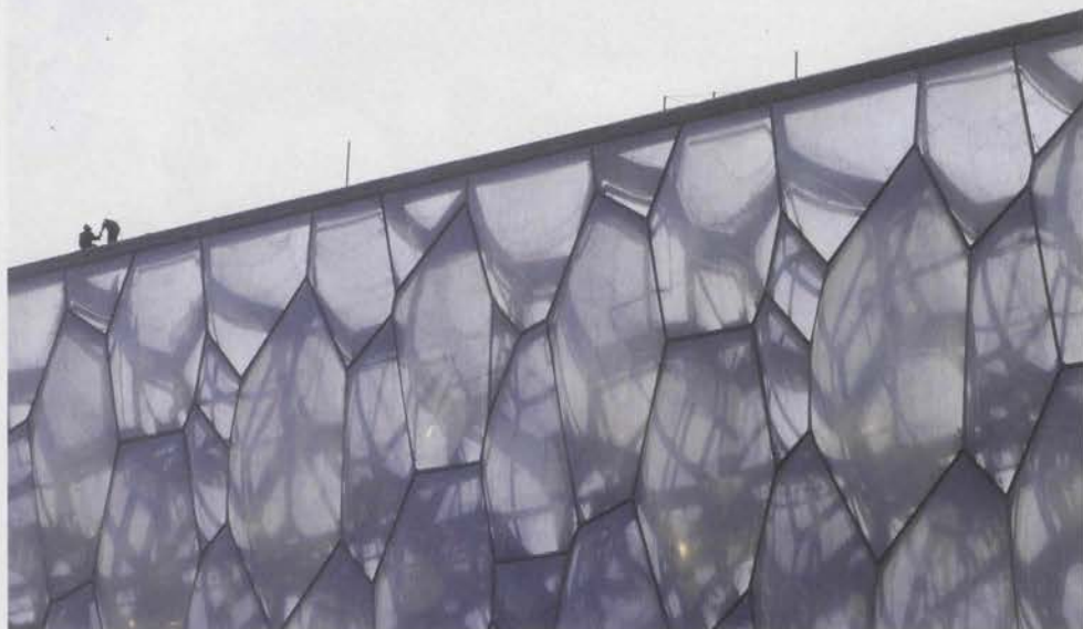
The "Water Cube" receives its exterior membrane. IC
