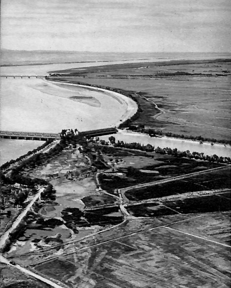
A hydro-junction in the upper reaches of the Yellow River.
