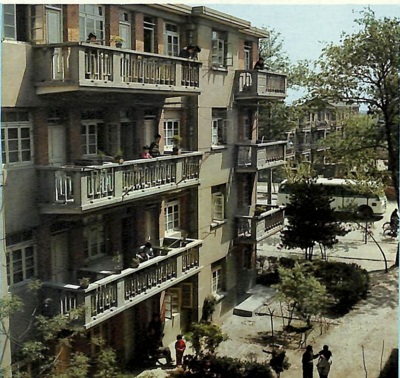
One of the newly-built workers' housing districts.
