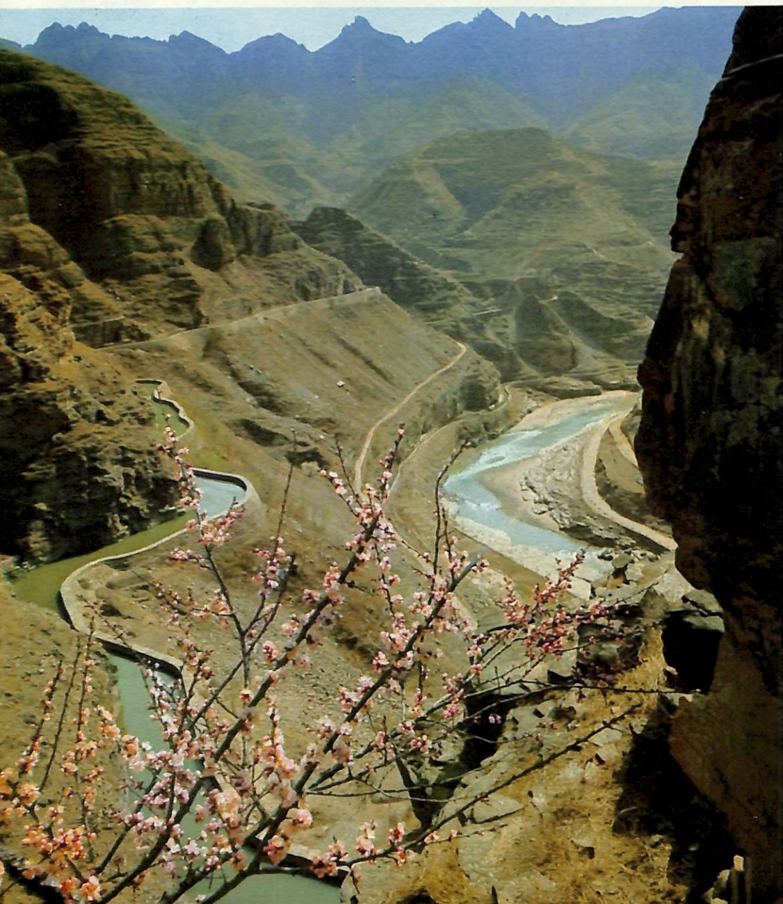
A section of the 1,500-kilometre Red Flag Canal built by the Linhsien people through their own efforts.
