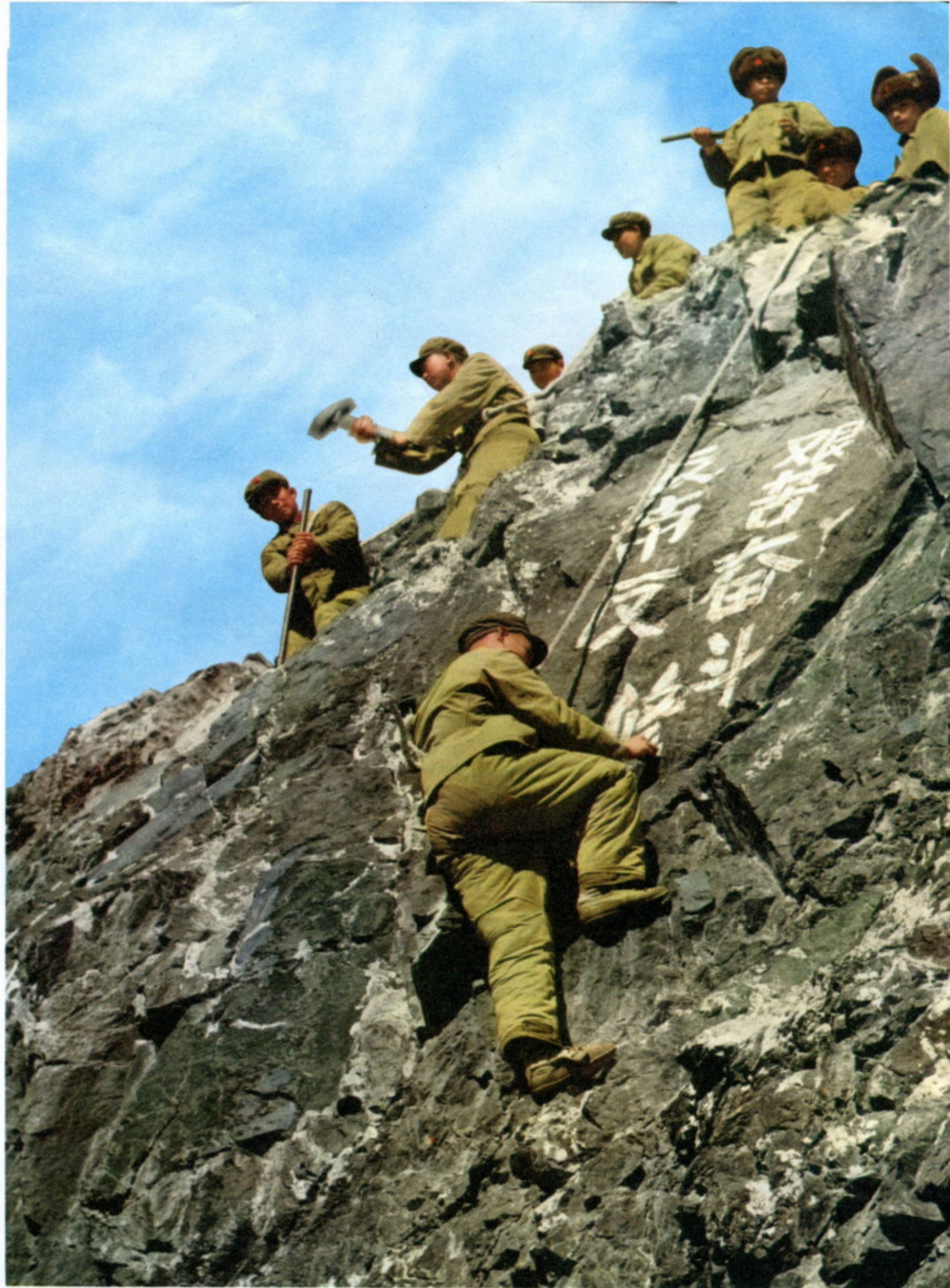
The construction site of arduous toil is also a battlefield against imperialism and revisionism. A fighter is inscribing the slogan, "Strive hard, oppose imperialism and revisionism", on a cliff.
