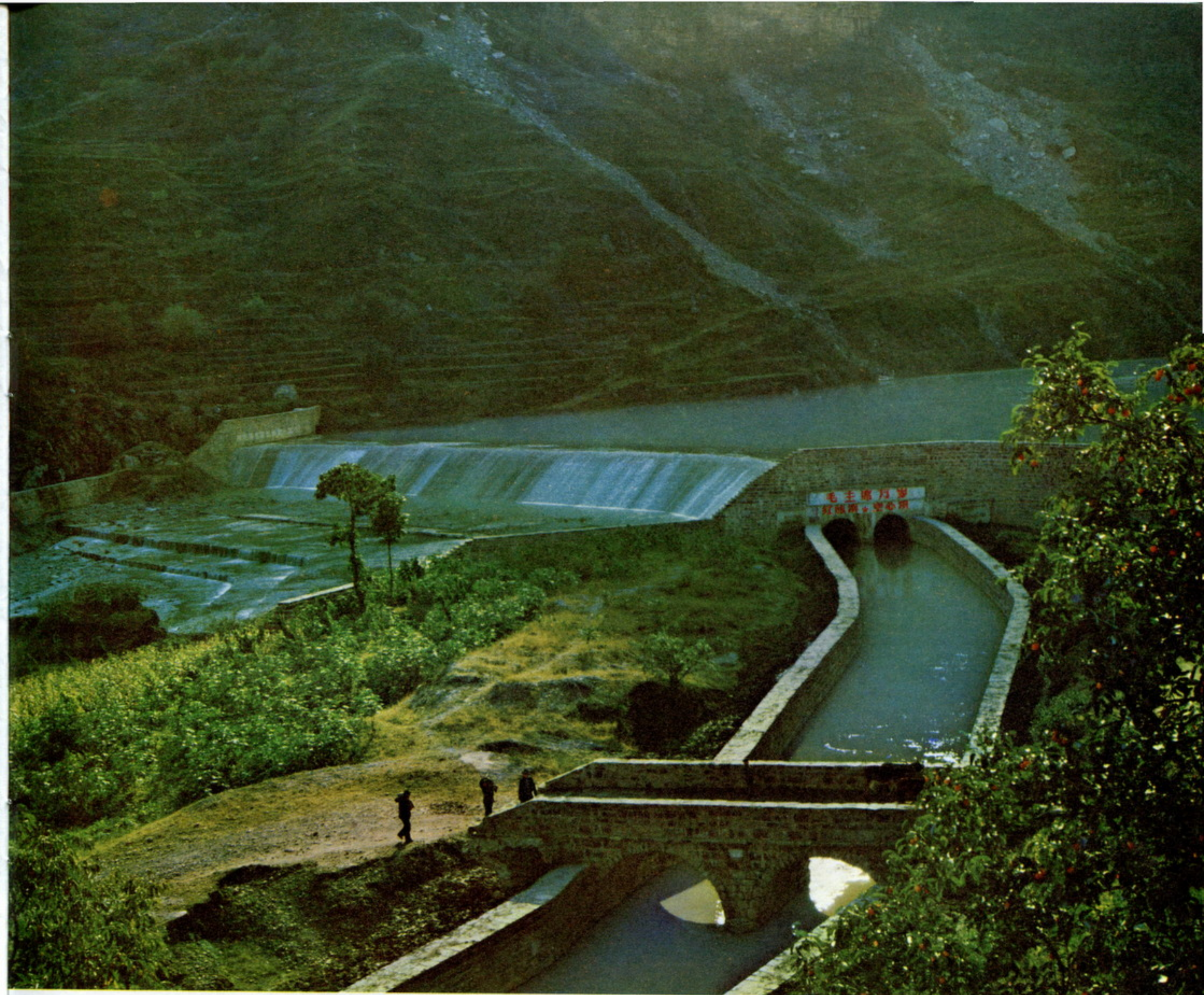
A dam with culverts — an important project in the construction of the "Red Flag Canal".
