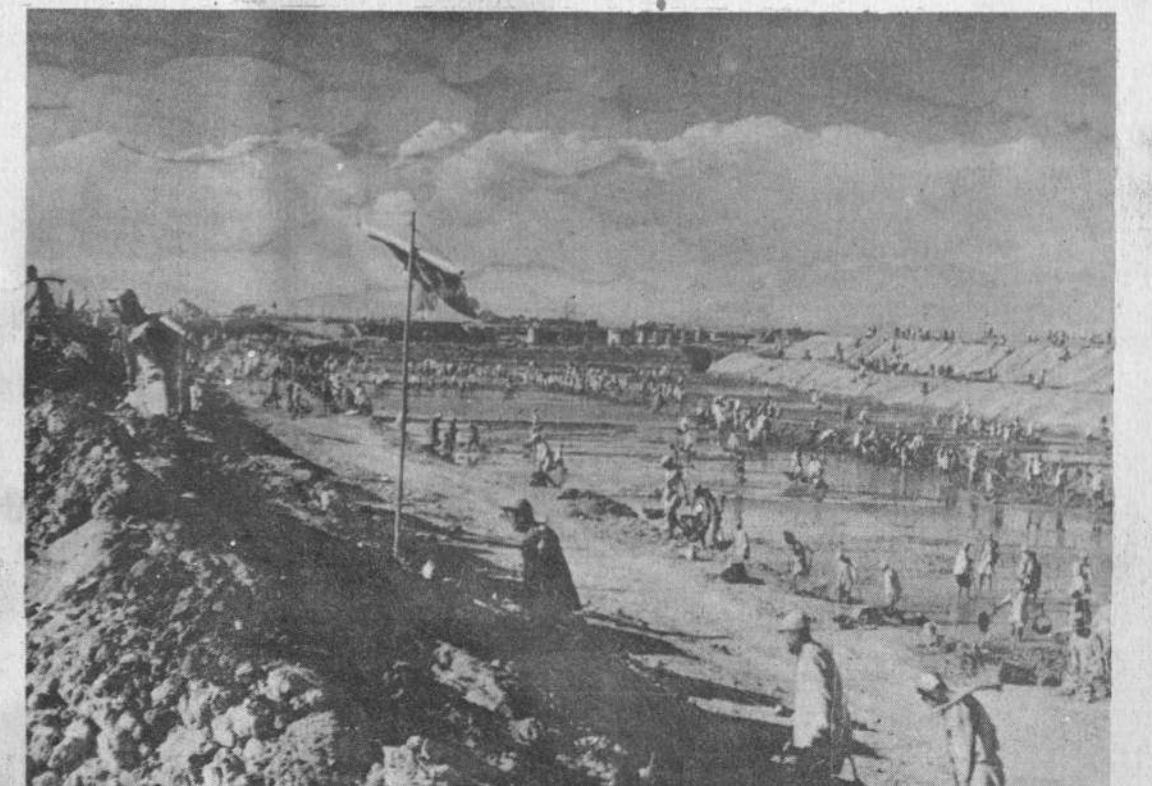
Hundreds of peasants take part in repairing the canal
