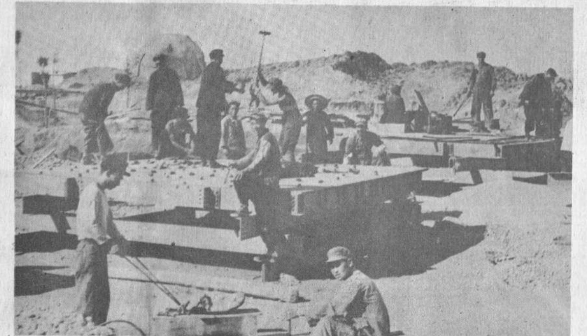
Installing the sluice gates
