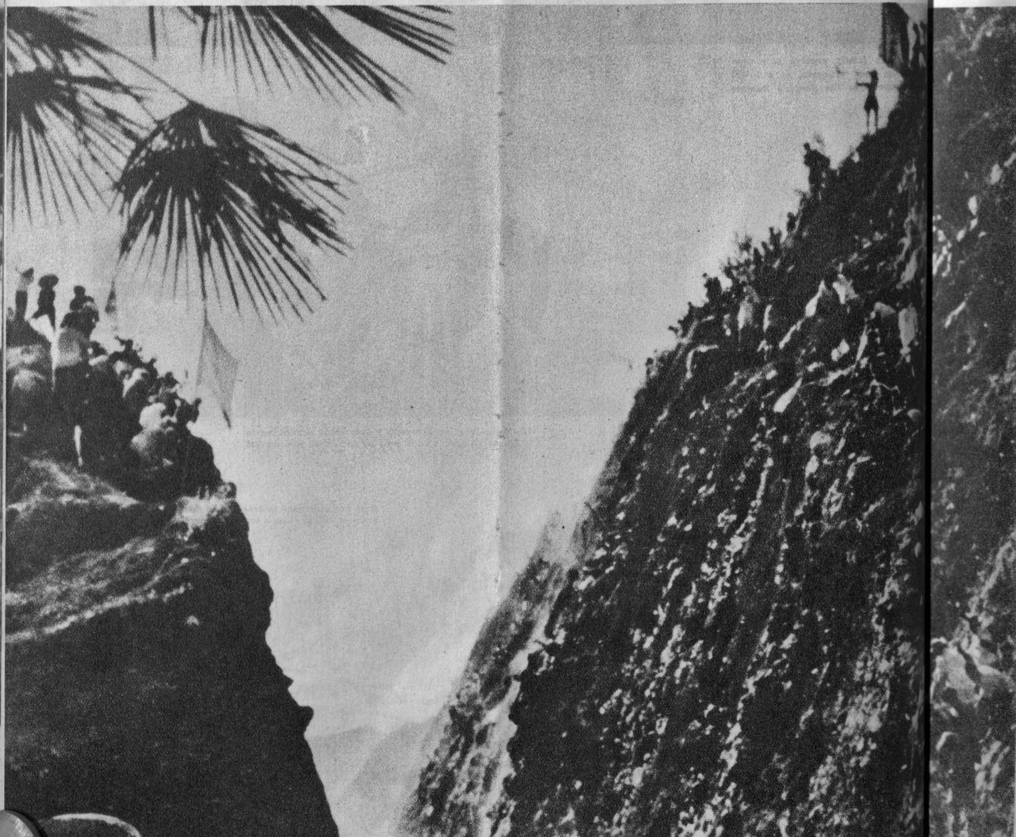
A deep railway-cutting through a mountain—illustrative of the engineering problems involved in carrying the railway through the mountainous areas of Szechwan Province
