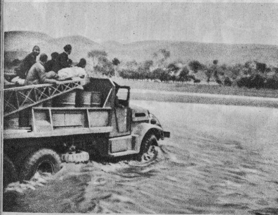
Equipment for the construction of the railway was transported both by train and lorry—in some places there were no roads, in others roads had to be built, but the supplies came through on time
