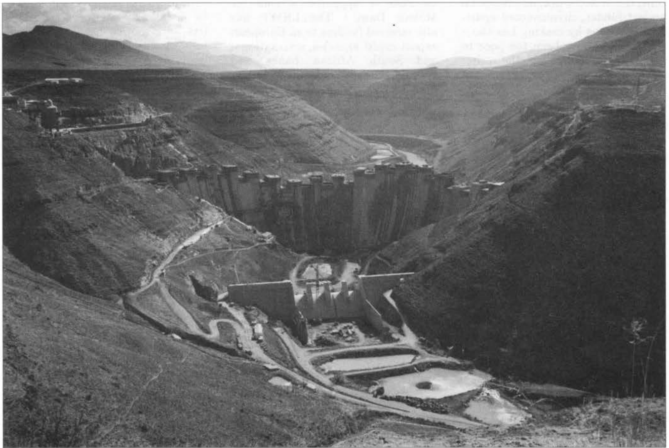
The 182 metre-high Katse Dam when it was under construction
