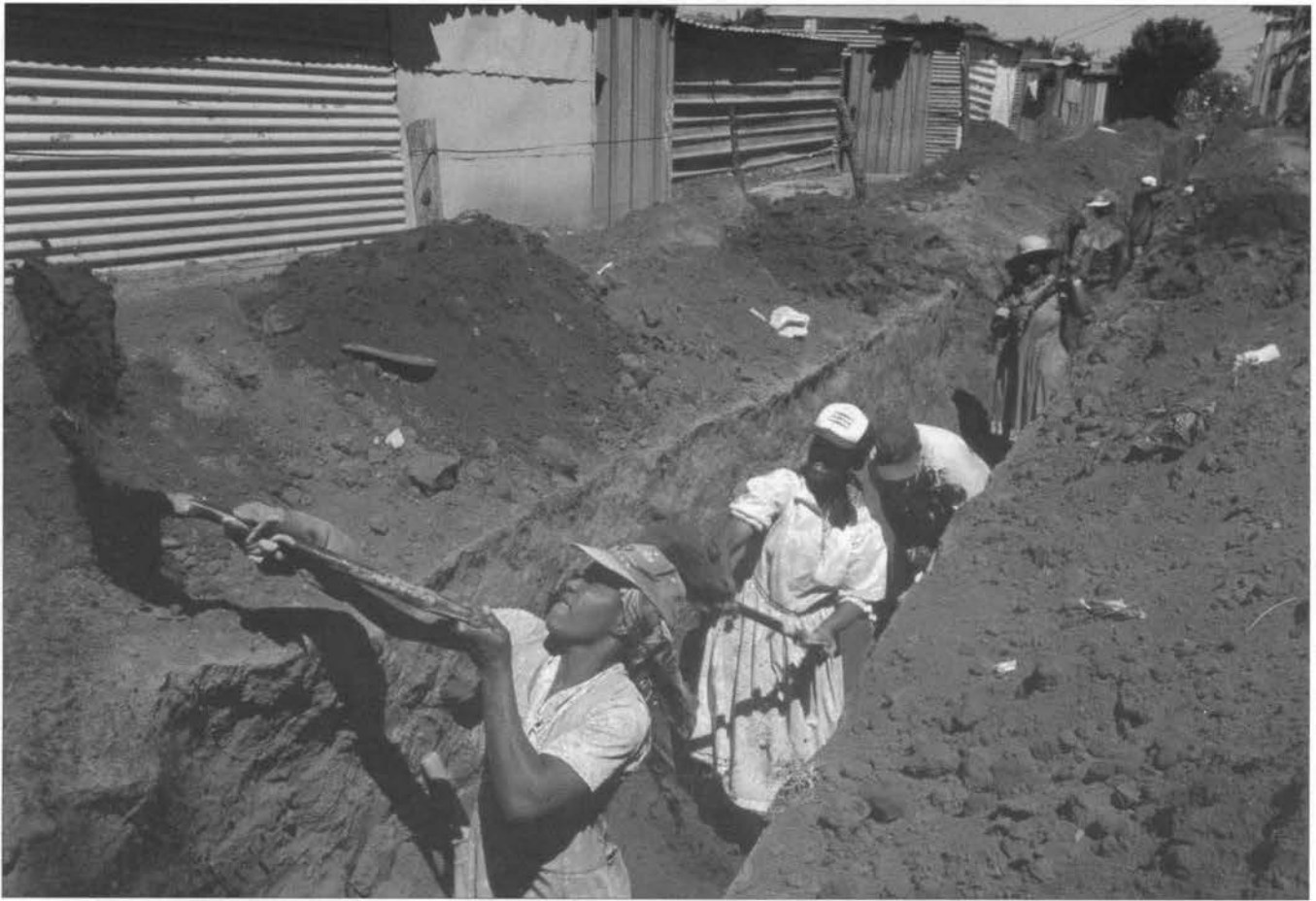
Constructing sewer system at Ivory Park squatter camp, east of Johannesburg
