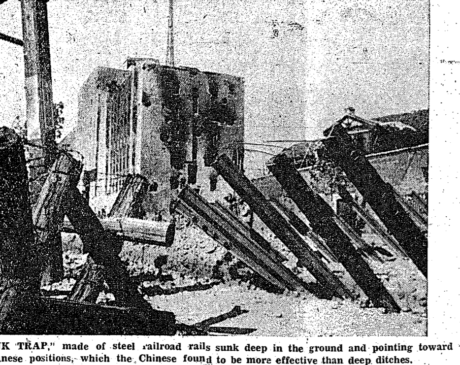
A "TANK TRAIN" made of steel railroad rails sunk deep in the ground and pointing toward the Japanese positions, which the Chinese found to be more effective than deep ditches.
