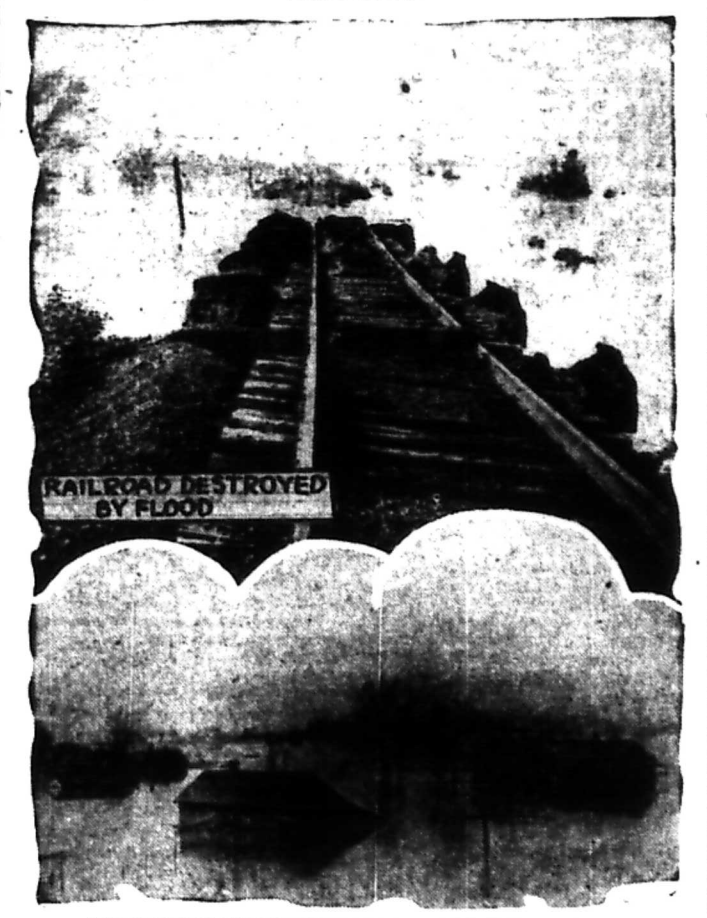
RAILROAD DESTROYED BY FLOOD
