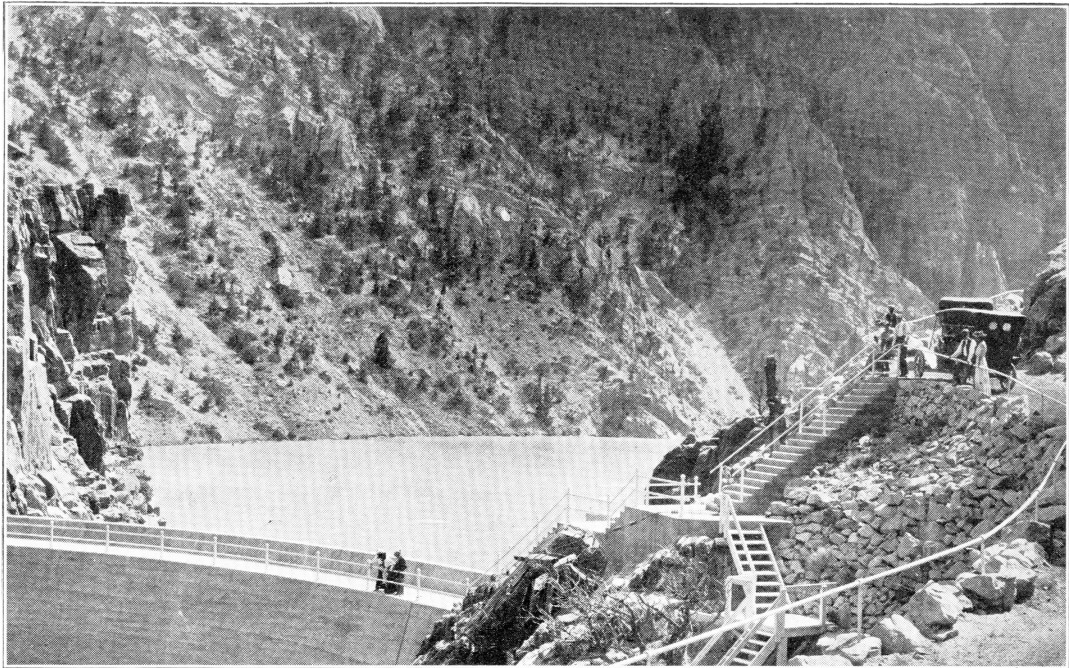
THE SHOSHONE DAM, CODY, WYOMING—ONE OF THE FACTORS WHICH IS RAPIDLY CHANGING THE OLD COW-COUNTRY INTO AGRICULTURAL AREAS. THIS DAM IS 329 FEET HIGH AND FORMS A LAKE 12 MILES LONG AND SEVERAL MILES WIDE.
