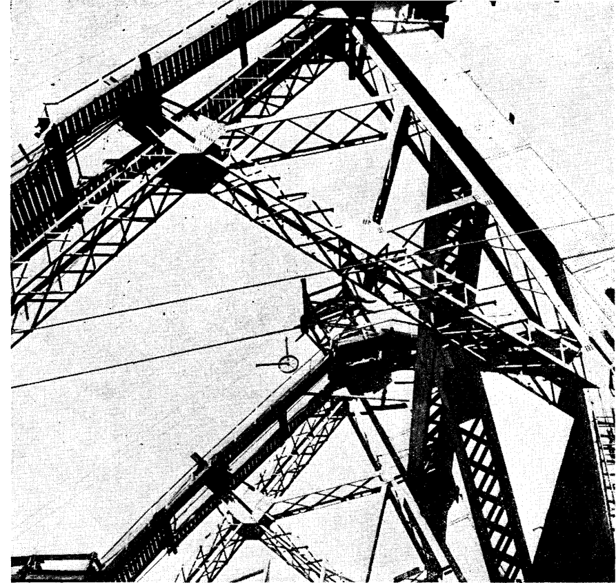
Riveting steel structures such as these on the Tri-borough Bridge meant lead poisoning for fifty workers.
