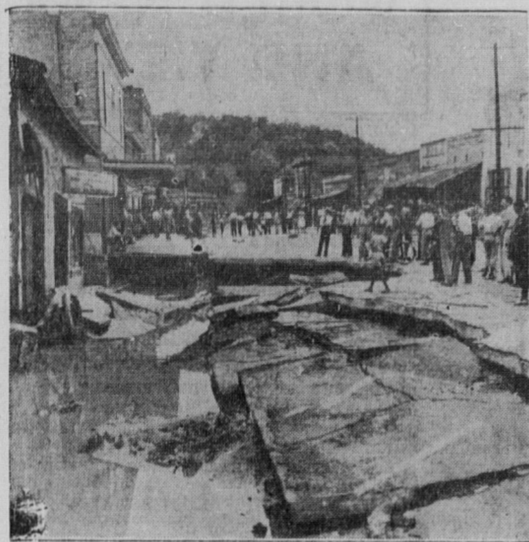
Undermined by overflowing waters from a swollen tributary of the Alabama River, this section of Prattville's main street collapsed. The flood was caused by heavy rains, forcing thousands of persons in the southern part of the state to flee their homes.
