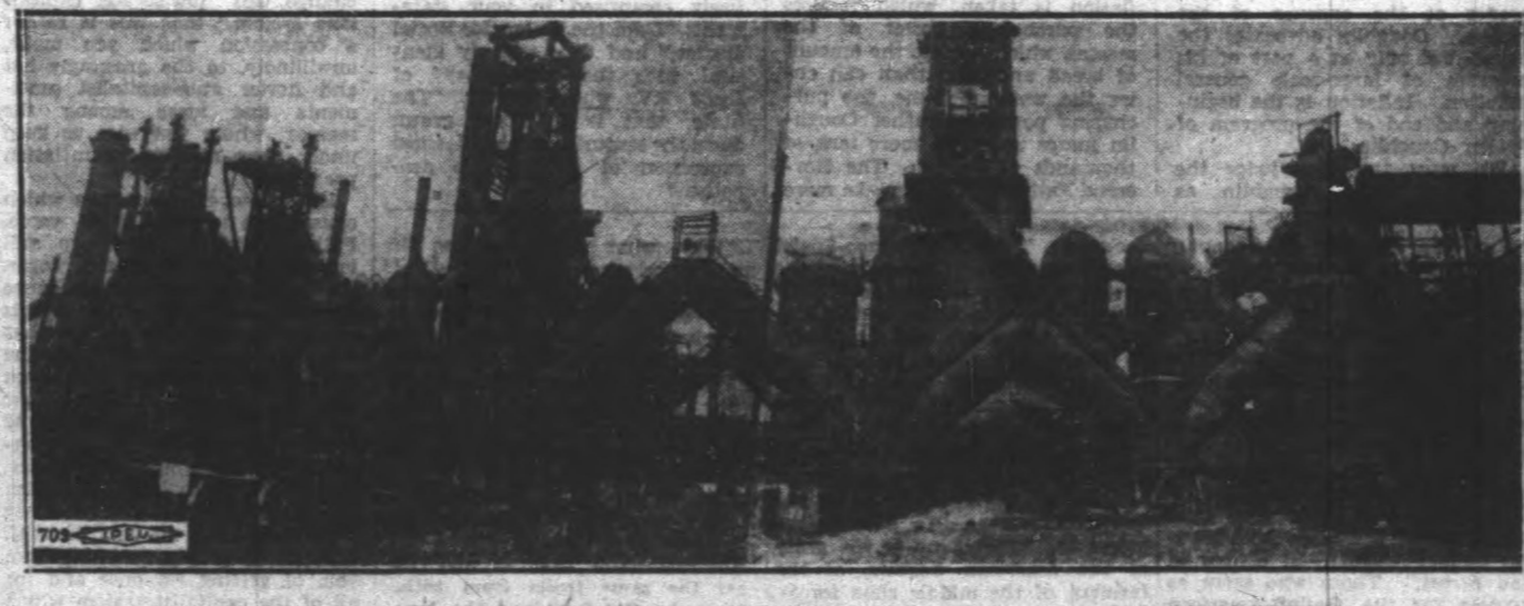
A HUGE UNIT OF THE STEEL AND IRON PLANTS AT MAGNITOGORSK
