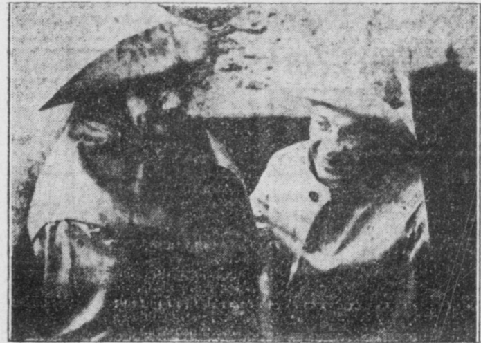
Here are two of the engineers in charge of the building of Moscow's projected subway, descending into a shaft ready to go to work. Moscow has grown tremendously with the moving of the capital there following the revolution and transport is a major problem. The subway is planned to help solve it.—(P. P. Pictures.)
