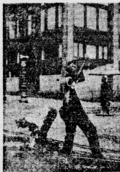
Negro Workers Repairing Street at Lowest Wage
