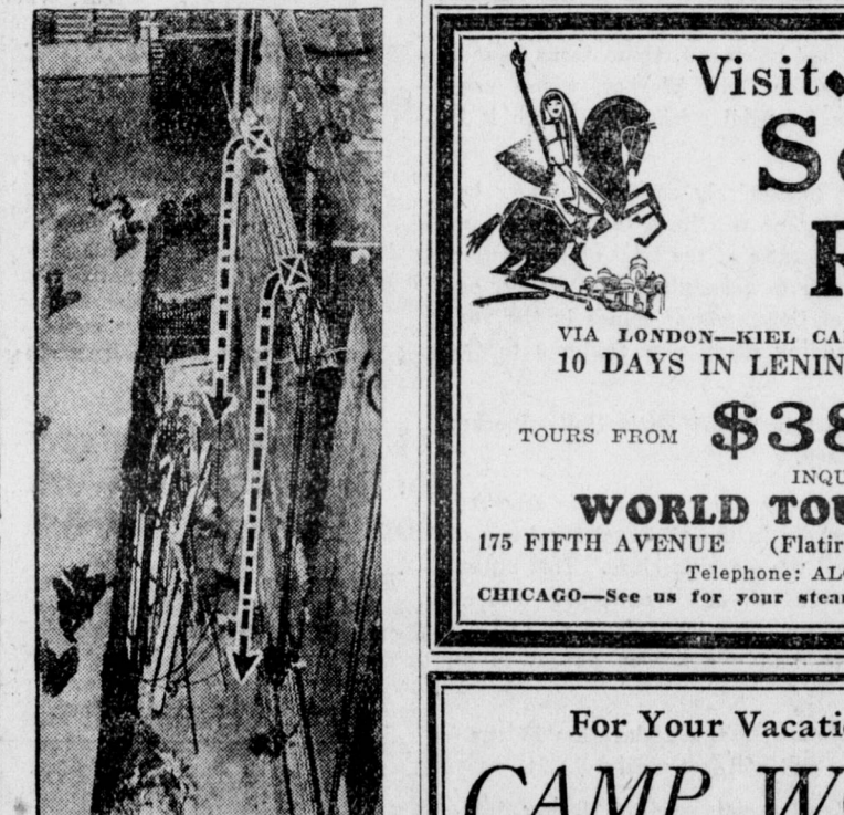
A swinging scaffold hoisted hastily on the Mariners Church threw two construction workers off their balance to instant death. Workers on the job say that elementary precautions by the contractors would have prevented the accident—but the boss was too busy calculating profits to think of such trifles as workers' safety.
