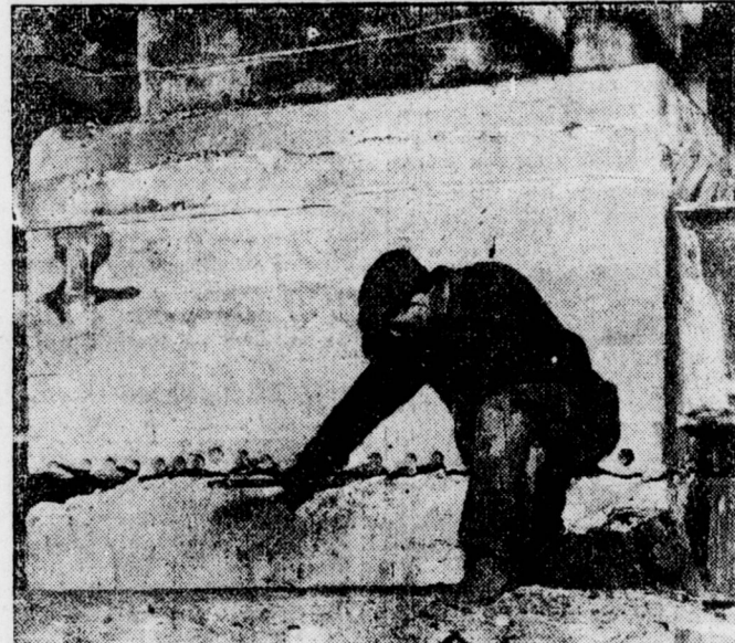
A job that required great risks on the part of the underpaid construction laborers was the raising of the elevated railroad station at City Hall, New York, an inch and a half. Photo shows one of the workers on this job. Accidents to workers, due to company neglect are frequent.
