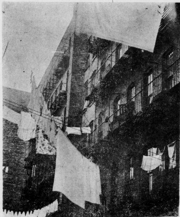
The rear of the row of tenements on Seventh Avenue, described today. Notice the iron balconies and the lack of stairways between them. They are supposed to be fire-escapes. —Photo by Nippon Camera Club.
