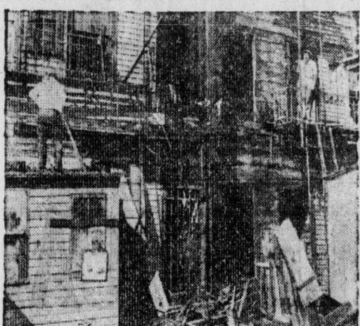
Fire in a shoe repair shop at Pitkin Ave. and Chester St., Brooklyn, menaced the lives of several workers and threatened to trap others in the contiguous block of frame buildings. It took hours for the firemen to get the blaze under control. Above, the ruins of the shoe shop.
