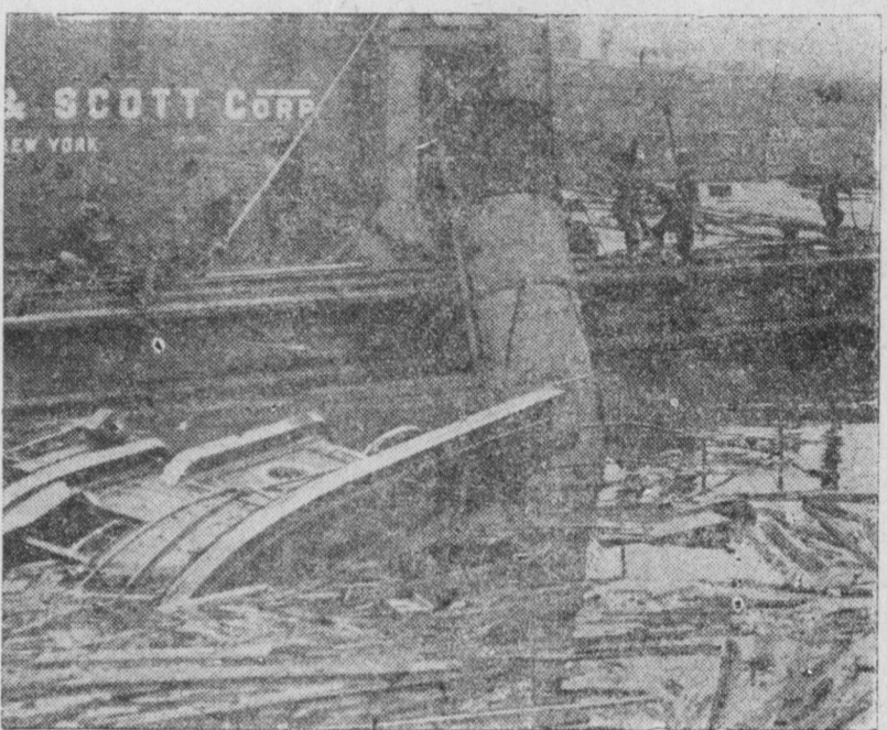
Deaths among barge and tugboat workers are a daily occurrence. Collisions and drownings take a heavy yearly toll among these men. The picture shows one sinking where the tugboat workers had a narrow escape. The tug in the picture, sank off pier 36 at the foot of Pioneer St., Brooklyn.
