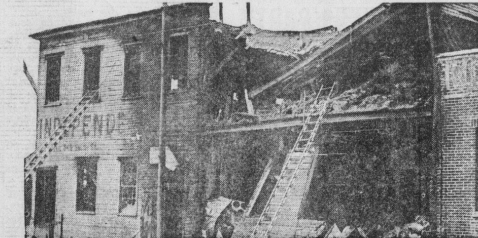
The picture shows the remains of what was formerly a varnish plant at 15 St. and 2nd Ave., Brooklyn. An explosion in a pulverizing machine caused the blow-up. Four employees barely escaped with their lives.
